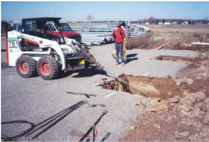
Concrete Breaker on Skid Steer
