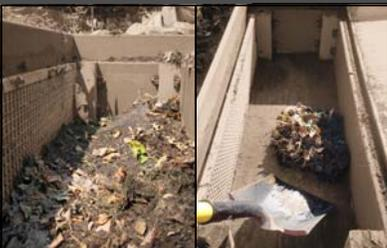
SEDIMENT, LEAVES, AND GRASS CLIPPINGS TRAPPED INSIDE THE CHAMBER ARE EASILY REMOVED BY THE LANDOWNER WITH A SHOVEL. THE DROP-IN FILTER WALL CAN BE EITHER SWEEPED CLEAN OR RINSED WITH A GARDEN HOSE TO MAINTAIN OPTIMAL FILTRATION CAPACITY.
