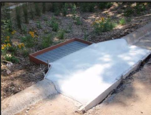
FILL VOID BETWEEN EXISTING CURB AND RAIN GUARDIAN. INSTALL FRAMING TO PREPARE FOR CURB-CUT AND APRON INSTALLATION. SIDES OF APRON SHOULD BE RAISED SIGNIFICANTLY TO BLEND INTO CURB AND MATCH TOP HEIGHT OF RAIN GUARDIAN SIDE DEBRIS WALL.
