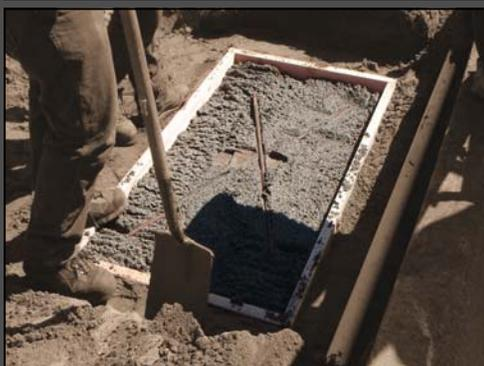
REBAR IS PLACED DIAGONALLY AFTER 2" OF CONCRETE HAVE BEEN POURED TO PROVIDE REINFORCEMENT OF THE CONCRETE BASE.
