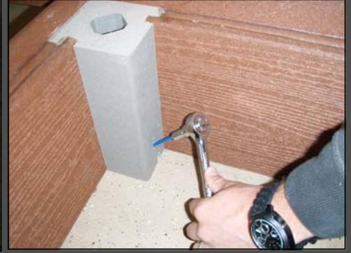
RAIN GUARDIAN PLACEMENT IS SET 26" FROM THE BACK OF THE EXISTING CURB. ENSURE THE CONCRETE BASE EXTENDS AT LEAST 4" BEYOND THE FILTER WALL TO SERVE AS A SPLASH DISSIPATER. APPLY ADHESIVE TO BASE OF RAIN GUARDIAN AND POSITION ON CONCRETE BASE. USE ADDITIONAL ADHESIVE AROUND BASE OF INTERIOR TO ESTABLISH WATER-TIGHT SEAL. USING PILOT HOLES IN CORNER POSTS, DRILL 3/16" HOLES INTO CONCRETE WITH 6 1/2" MASONRY BIT AND HAMMER DRILL. SECURE WITH 1/4" X 5" MASONRY SCREWS (PROVIDED).
