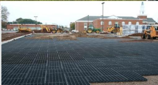
The **GEOBLOCK®5150** turf protection system is installed over a prepared 4-inch base course to support vehicle loading, protect the topsoil & vegetative root zone, and increase surface infiltration.
