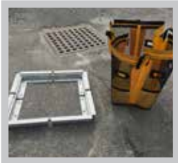
Insert the frame into the drop inlet.
